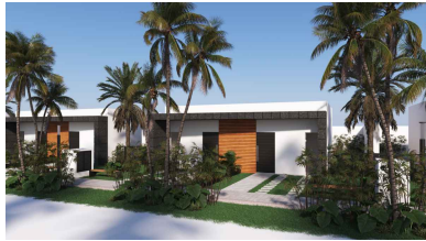
FACHADA PRINCIPAL/MAIN FACADE
