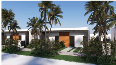
FACHADA PRINCIPAL/MAIN FACADE
