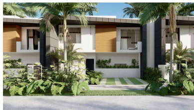
FACHADA PRINCIPAL/MAIN FACADE
