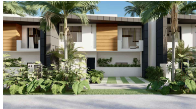
FACHADA PRINCIPAL/MAIN FACADE
