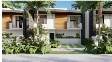
FACHADA PRINCIPAL/MAIN FACADE
