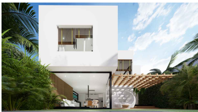
FACHADA POSTERIOR/BACK FACADE
